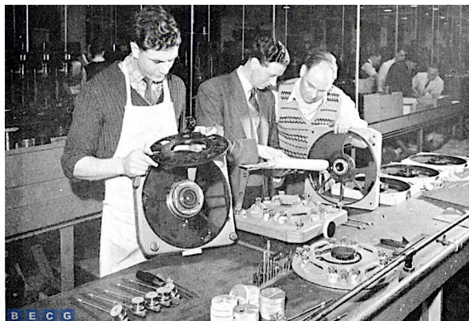
Lens turret assembly in Section 15. J. Warner, chargehand centre, with R. Wood, right, who is fitting turret bearings, and G. Murdy, left, fitting the filter ring 'The Marconi Companies and their Peoples', Vol 6, No. 7 February 1956 p18
