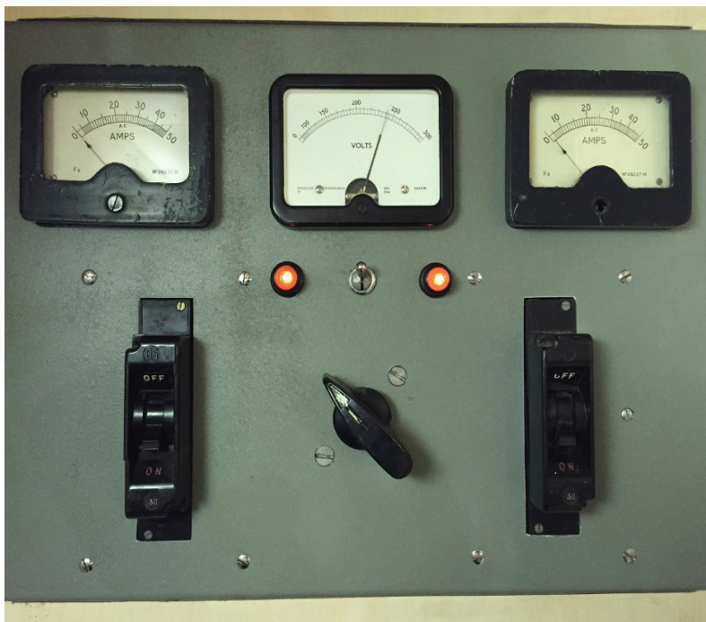
Control panel for automatic voltage regulator, affectionately known as Claude because it was made by Claude Lyons
