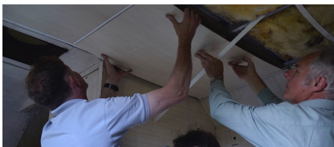
Formica and fibreglass fitted by Martin and Richard.
