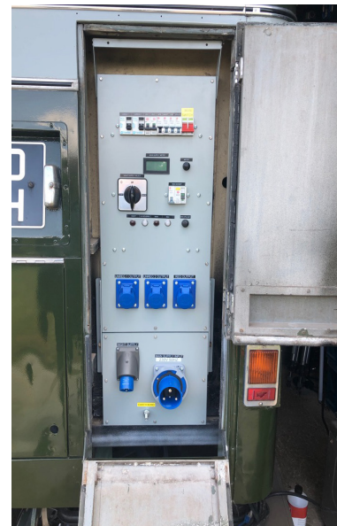
Vivat mains intake panels, old and new. Richard designed and built the new panel.
